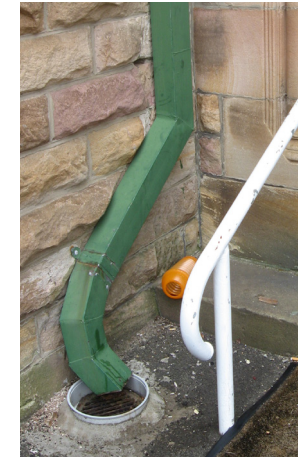
Figure 2.16 Stonework cut to accommodate downpipe, and later handrail
