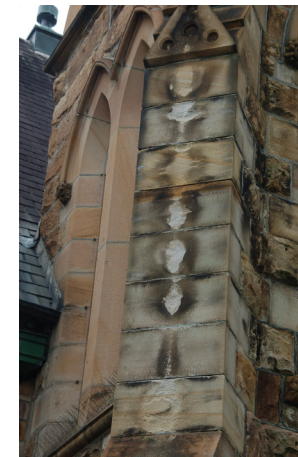
Figure 2.12 Typical buttress with typical deterioration of sandstone
