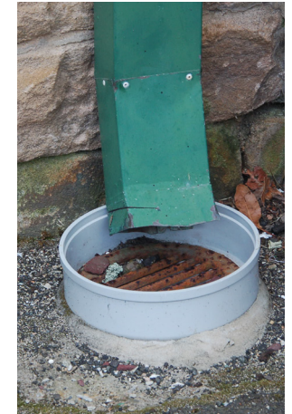
Figure 2.17 PVC collar of downpipe drain
