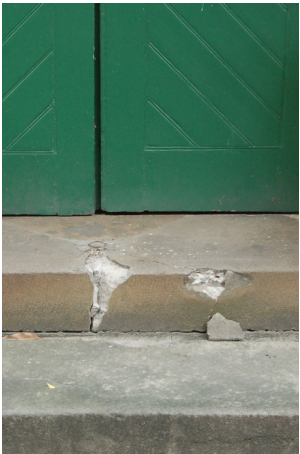
Figure 2.18 Examples of damage to stonework due to wear and tear (left) and past work (right)
