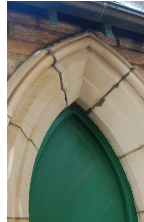
Figure 2.20 Example of inappropriate pointing
