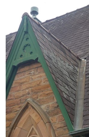
Figure 2.5 Typical gable and timber infill (with missing element on left), slate shingling, ridge vent and valley gutter
