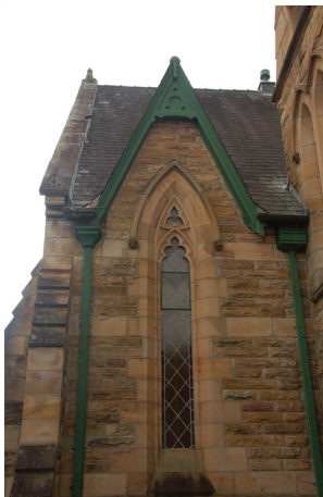
Figure 2.7 Typical lancet window and gable with recent leadlight
