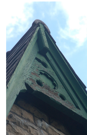
Figure 2.6 Deteriorating gable infill
